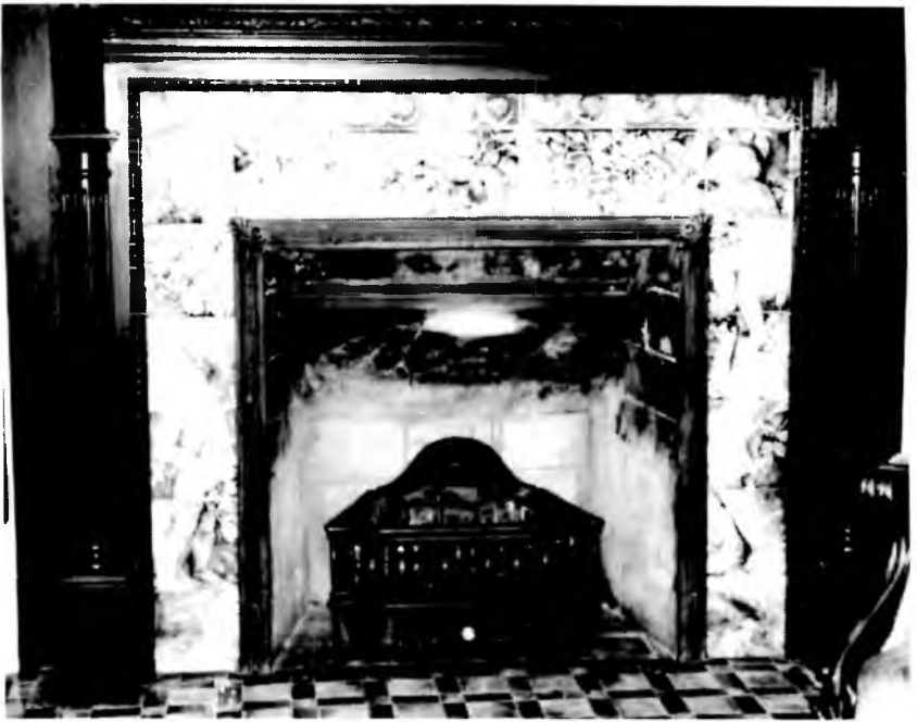
Figure 2: Fireplace showing tile detail.
