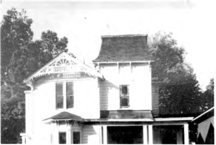
Note: All photographs are by Harvie P. Jones, FAIA. Courtesy of Lynn Jones. Figure 1: East front, Goldsmith-Donovan House, as it looked in 1996.
