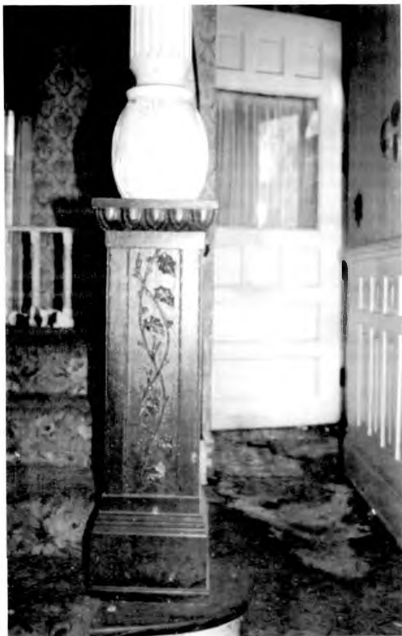
Figure 7: Detail of staircase, December 1996, before removal of black and white paint.
