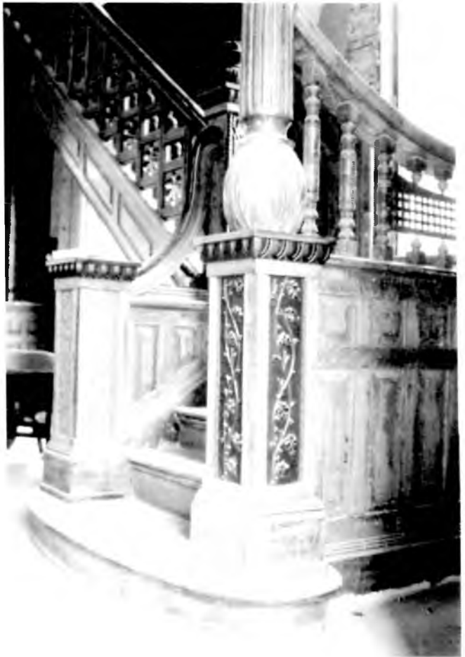
Figure 8: Staircase during cleaning, December 1997. Some of the black paint remains.
