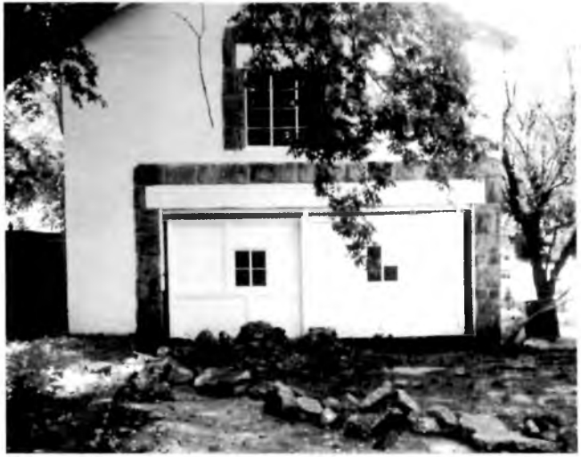
420 Newman garage before renovation—The block and stone structure was built by the Pizitz family in the 1940s to match the home and offer a rentable apartment. The renovation retained and expanded the apartment and storage space. Photo courtesy Raymond Hamilton, Jr.
