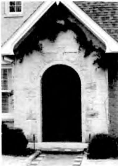
Restored front entry porch of 420 Newman—The front door was moved back to its original location, opening the small recessed entry porch. The multi-colored tiles line the walk to the street. Photo by Carol Roach.
