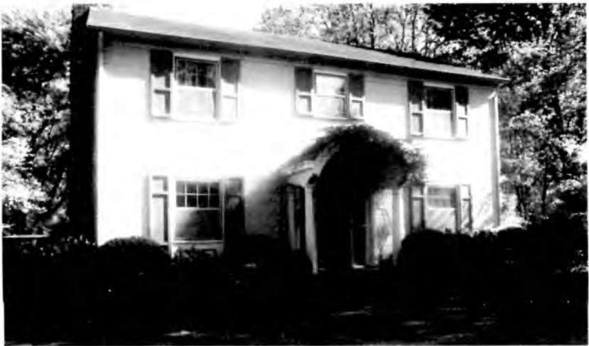
412 Newman Avenue—The colonial revival facade of the symmetrical house includes wide plank siding, dentil molding under the eaves, a Federal style entry door with fan and sidelights as well as an arched and stepped bracket porch resting on simple Doric columns. The curved herringbone walkway in brick echoes the brick of the chimney. Photo by Cynthia Parsons.
