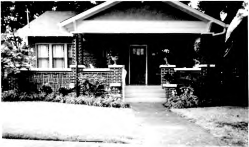
436 Newman Avenue—The red brick bungalow of Donna and Michael Costellano is typical of the Newman Avenue homes built in the late 1920s. The wide overhangs, the shallow front peak and the brackets supporting the porch roof over brick piers and stepped porch wall reinforce the horizontal facade. Photo by Donna Castellano.
