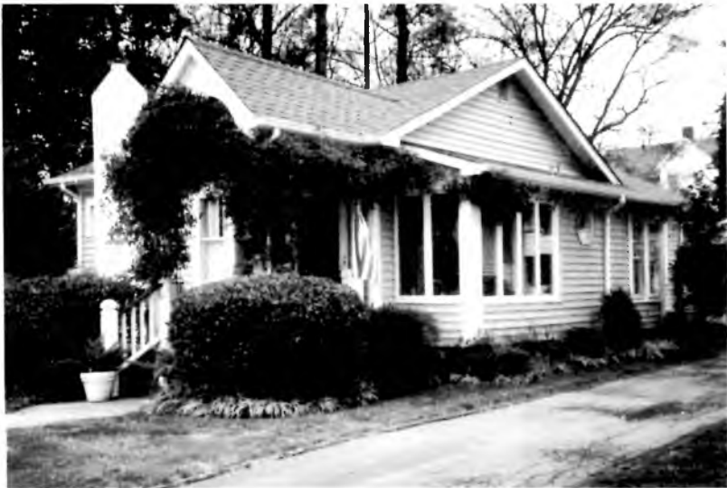
Site of original entry—The original side porch and entry after renovation. The overhang, interior beadboard and siding, and dimensions of the porch remain but are enclosed to create a sunroom and additional bath and closet space. Photo by Carol Roach.
