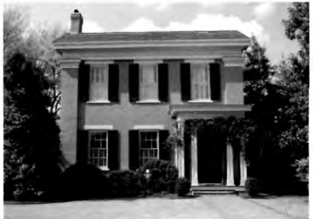
413 Randolph Avenue, Greek Revival, ca. 1851
