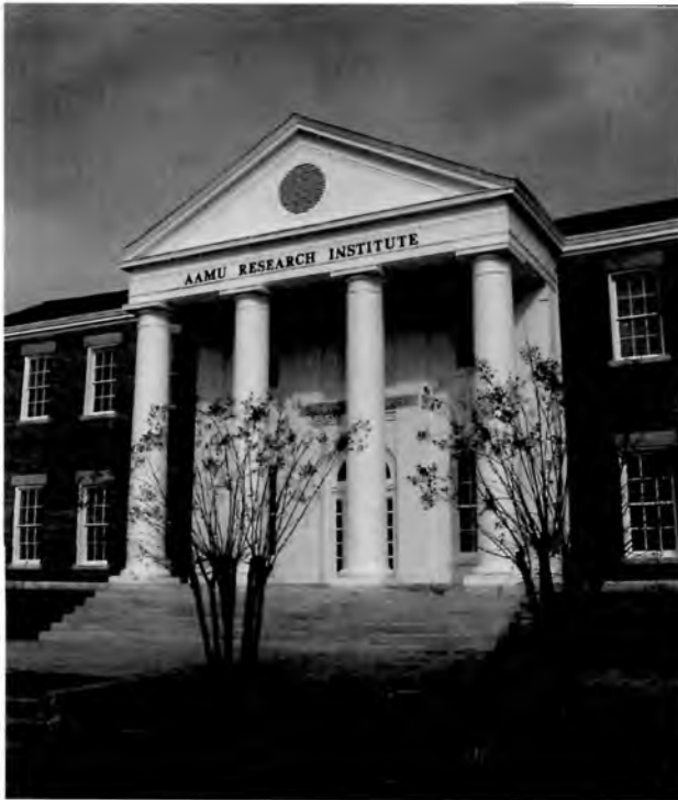
Old Carnegie Library, Alabama A&M University, 1904 and 1946 Courtesy SKT Architects
