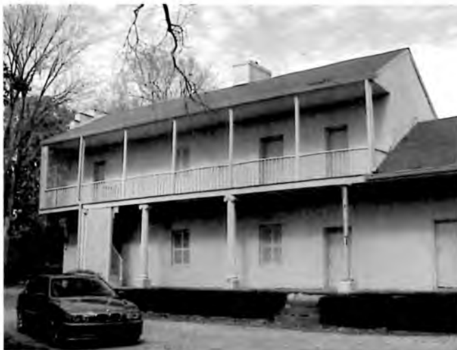
West side view of upper and lower galleries. Ionic columns were probably salvaged from demolition of original house, around 1900.
