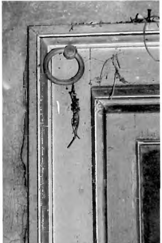
Typical Federal window and door casing. This profile is found in all rooms except the upstairs center room and the smokehouse.
