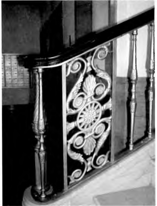
Mezzanine balustrade with lyre + sunburst + inverted lyre pattern, 2004. Hotel mailboxes in background. Courtesy Fuqua Osborn Architects. Missing in this photo is the brass ball that topped the newel. Every time someone discovered that the ball was removable, it would go missing for awhile. See the wedding reception photograph in this issue (page 44) to view both balustrades’ newel toppers in their proper places.
