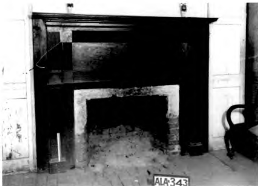
Mantel and flanking cupboards in second-floor east room. Historic American Buildings Survey, Alex Bush, photographer, May 21, 1935
