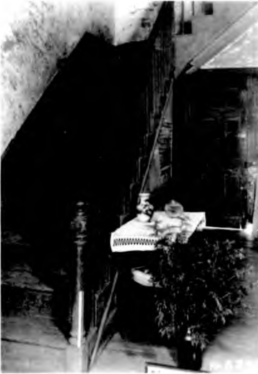
Stairs on west side of entry hall. Historic American Buildings Survey, Alex Bush, photographer, May 21, 1935
