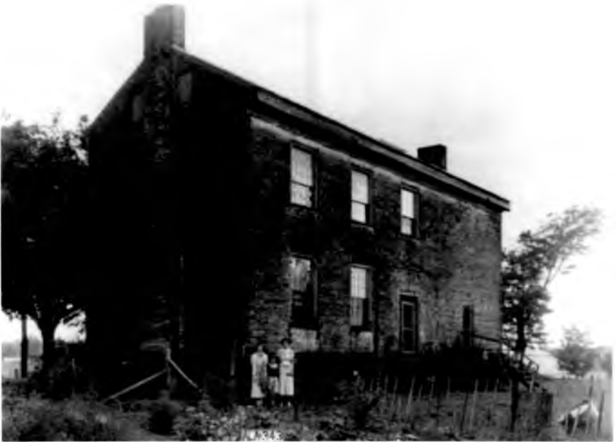
Cotton Hill in 1935 showing the north-facing rear and east side elevations. Historic American Buildings Survey, Alex Bush, photographer, May 21, 1935
