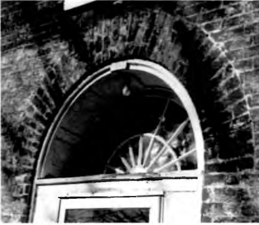
Front entry fanlight and brickwork of Cotton Hill; doorway infill is not original. Photograph by Harvie Jones, F.A.I.A., 1981. Courtesy Architectural Collection of Harvie P. Jones, University of Alabama in Huntsville
