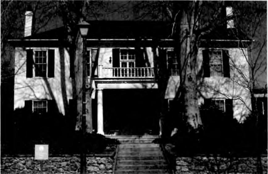
The house at 621 Franklin Street began in the 1820s as two rooms and a stair hall and was expanded during the later Federal period to nine rooms. Photograph by Linda Allen, 2006
