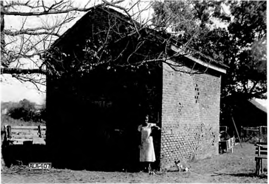
The importance of the smokehouse can be inferred by its proximity to the rear of the main house. This brick example from New Market illustrates a common local design with a vertical-plank door, diamond-patterned vents on each wall, and front gable roof. Photograph by Alex Bush for HABS, 1935
