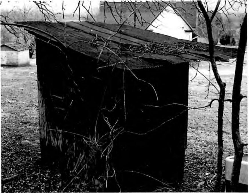
This Jackson County privy, still standing but abandoned, illustrates a primitive example of a necessary house; a sloped roof to keep off rain, one small window for ventilation, and an opening in the bottom of the rear wall to facilitate cleanout. Photograph by Linda Allen, 2005
