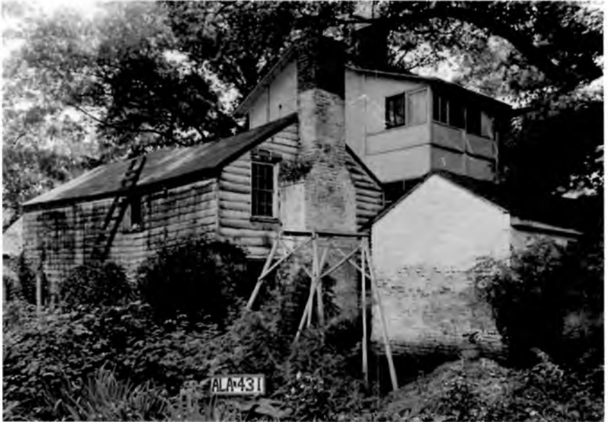
A rear view of the Cabaniss outbuildings as they appeared in 1935. The small brick structure on the right contained the dairy and well house; the larger two-story frame structure was the kitchen, slave quarters, and smokehouse. Demolished. Photograph by Alex Bush for HABS, 1935
