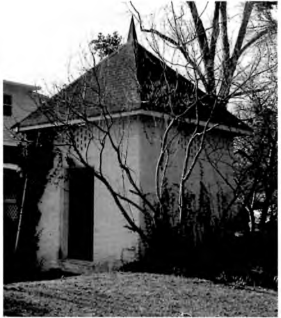
This extant smokehouse behind the house at 609 Adams was constructed in the 1870s, which may account for its reduced proportions. Although the main house was of frame construction, the smokehouse was brick and topped with a pyramidal roof and finial. Photograph by Doug Brewster, 2004
