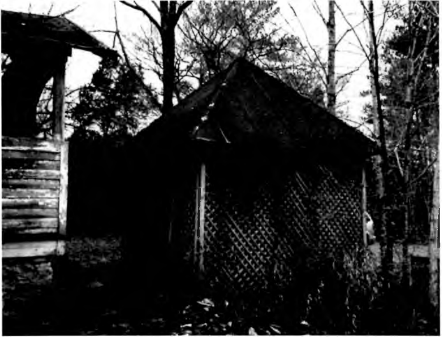
This well house on Jeff Road was located just feet from the kitchen; its square shape, pyramidal roof and latticed walls are characteristic of many such dependencies. It and the house were burned in 2003. Photograph by Linda Allen, 2003
