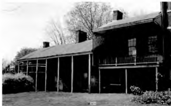
In 1934, the 518 Adams house was documented in drawings and photographs by HABS. The two-story section on the far left provided living spaces for house slaves, the adjacent section without a balcony but with the largest chimney would have been the kitchen, and the taller two-story section on the right provided access to the house and dining room. Photograph by W. N. Manning for HABS, 1934
