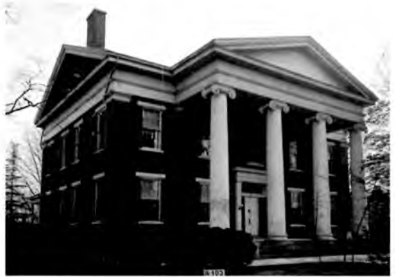
The Bibb-Hutchens house at 300 Williams Avenue as photographed in 1934 by W. N. Manning of the HABS team
