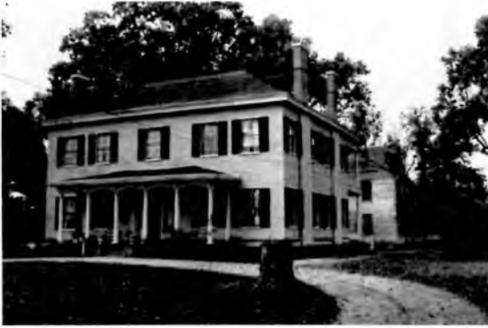
Quietdale, south front, a house that preservation architect Harvie P. Jones described in his Quietdale photograph book as showing “3 period influences in one: Fed. shape; Greek Revival interior details; Italianate porches (not original).” Slave quarters partially visible at rear. Photograph by Harvie P. Jones, FAIA. Courtesy Ira and Billie Jones
