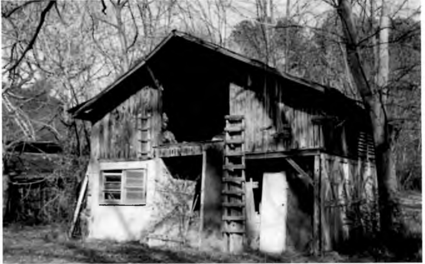
Nearby carriage house/barn showing alterations for changing uses over the years. Photograph by Linda Allen, 2004.
