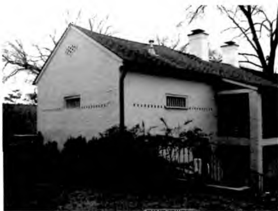
The south end of the kitchen building contained the smokehouse and displays a typical diamond-shaped ventilator in the end wall required for proper smoking of meats. Photograph by Lynn Jones, 2006
