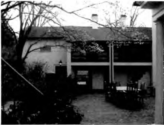
The kitchen dependency is seen here after its renovation by Rhett and Melanie Murray. The exterior cooking fireplace referred to is located in the ground floor breezeway which is visible here beneath the upper gallery. Photograph by Lynn Jones, 2006
