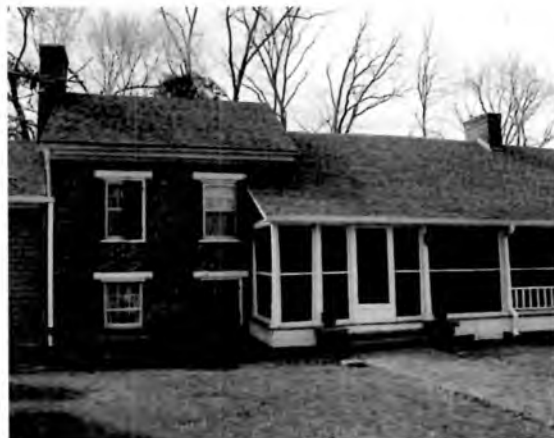
A side view of the McCrary-Thomas house illustrates three separate phases of construction, with the oldest, two-story section in the center, the replacement house dating from the late 19th century on the right, and the most recent, a frame addition, on the left. Photograph by Ralph Allen, 2006
