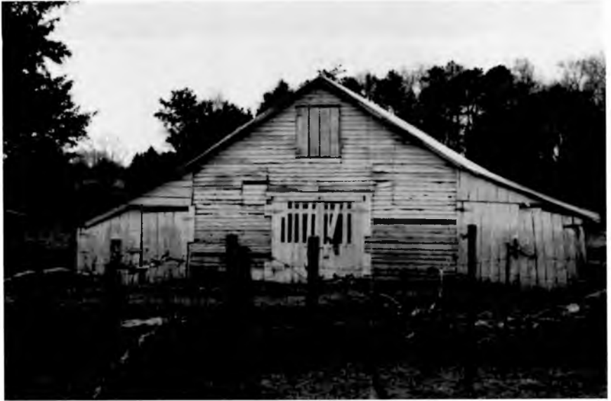
The McCrary-Thomas property still retains two barns, which probably date from the late 19th century. This is the smaller one and like the smokehouse has had a small shed added to each side. It continues the tradition of building farm dependencies to a rectangular plan with gable roof and entries under the gables. This is the smaller of the two barns and was once whitewashed. Photograph by Ralph Allen, 2006
