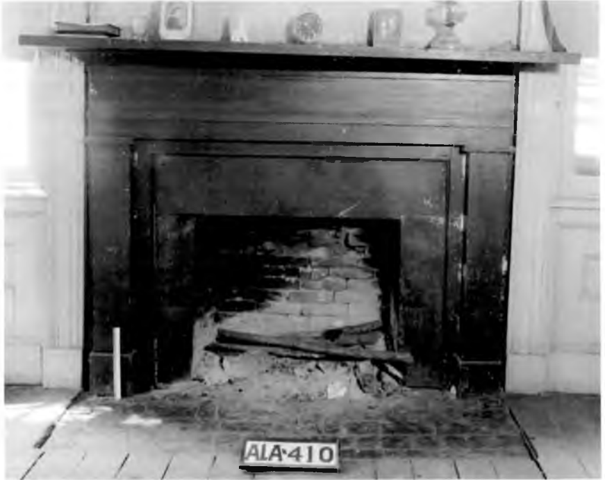
The only interior shots of the Horton house are of two fireplaces, neither of which had been altered to burn coal as were so many in the late 19th century when it became commercially available. Photograph by Alex Bush for HABS, 1935
