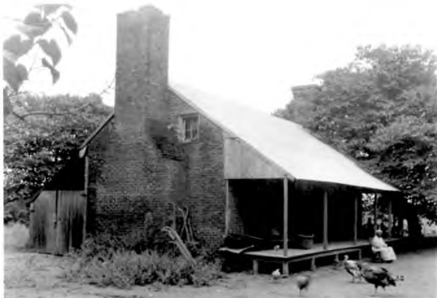
This two-room, brick structure behind the house reputedly was the original kitchen and dining room. Photograph by Alex Bush for HABS, 1935
