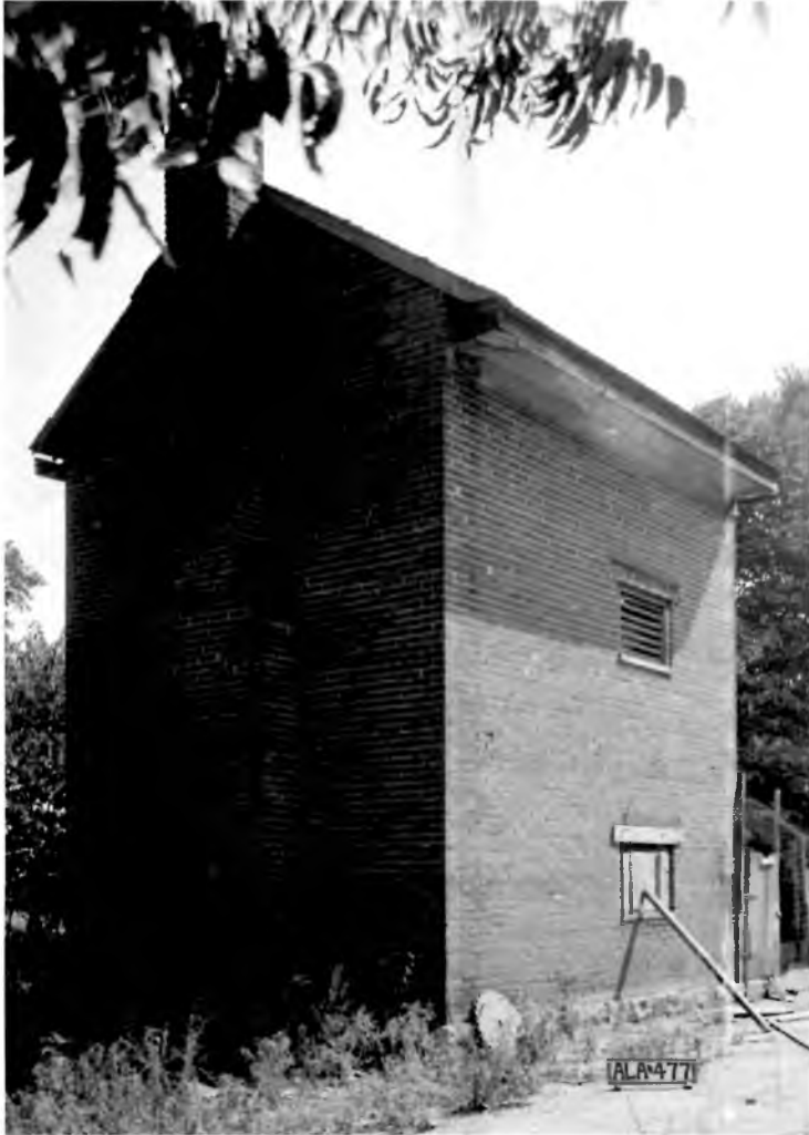
Built to the same massive scale as the house, the smokehouse still stands today in excellent condition. A huge fireplace on the ground floor produced smoke to preserve the meat, which was hung from rafters on the upper level. The small, louvered side vents now have glass installed behind them. Photograph by Alex Bush for HABS, 1935
