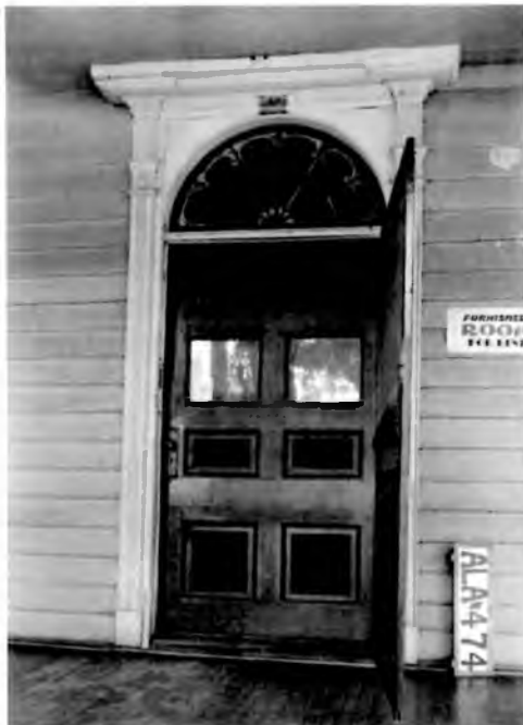
Detail of the Federal doorway with fanlight. The sign advertises, "Furnished Room For Rent." Photograph by Alex Bush for HABS, 1935
