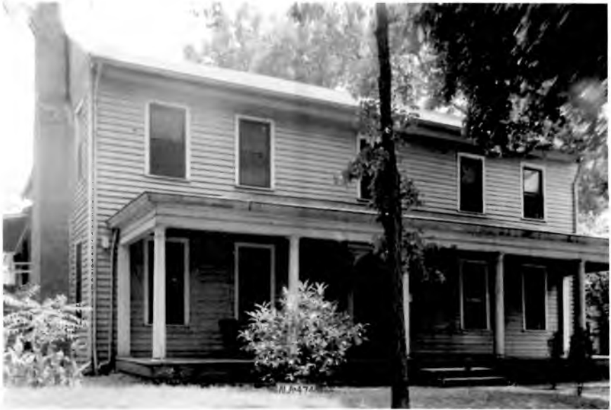
After its 1908-1913 conversion to a boarding house, the dwelling gained a new porch that extended the width of the façade. Photograph by Alex Bush for HABS, 1935
