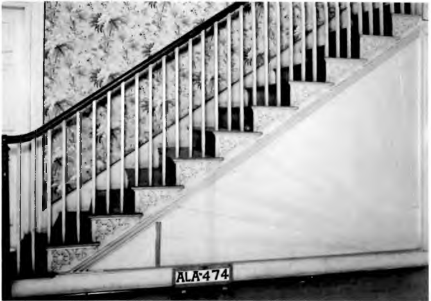
Fan detail on staircase. Photograph by Alex Bush for HABS, 1935
