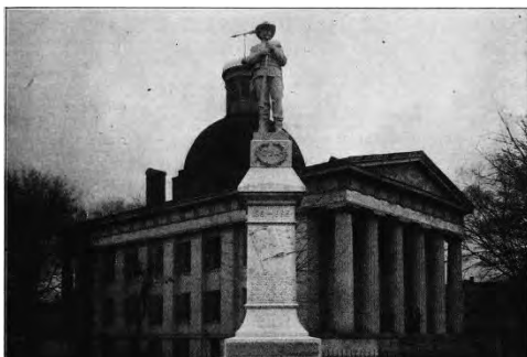
In front of the 3rd Madison County Courthouse.
